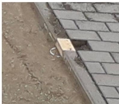
Side post foundation formwork
