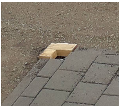
Goal post foundation formwork
