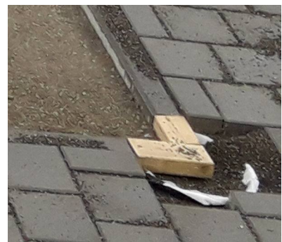
Corner post foundation formwork
