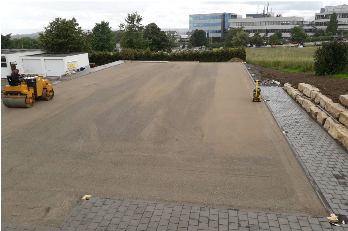
Gravel layer level and evenly compacted, firm and shear-resistant
