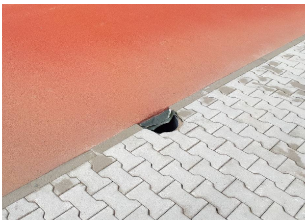
Installed synthetic surface
