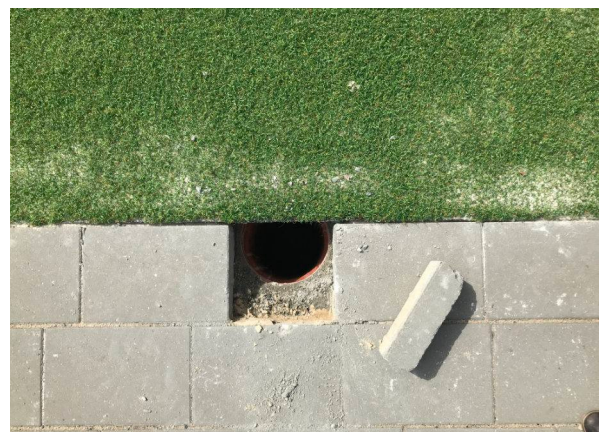
Installed artificial turf
